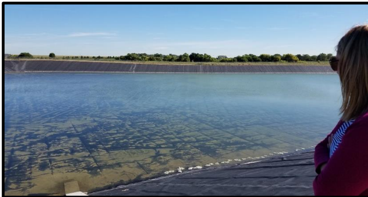
Irrigation Water Storage Lagoon
