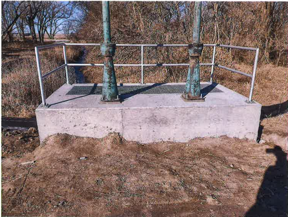
West Point Levee Improvements Construction: Gatewell Structure Raise at Sta. 98+19
