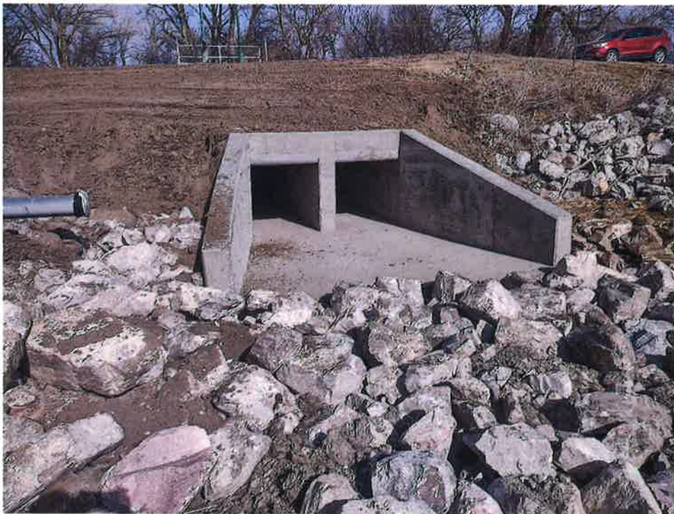
West Point Levee Improvements Construction: Box Culvert Extension at Sta. 57+26
