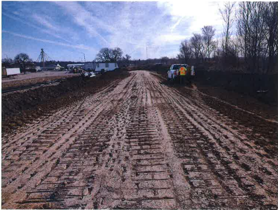
West Point Levee Improvements Construction: Sta. 123+00 Looking East
