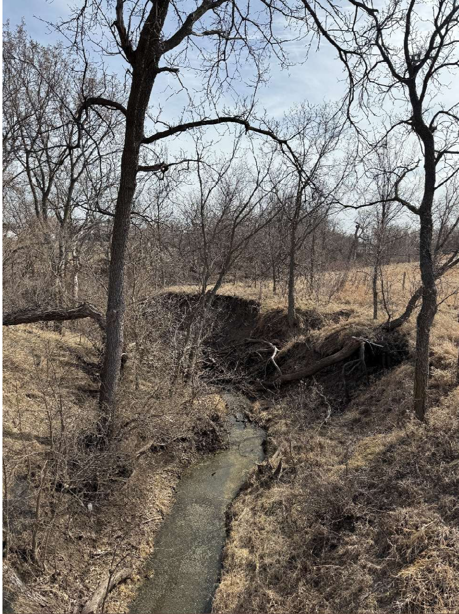
Figure 8. Existing Springfield Creek bank failure immediately downstream of MOPAC Trail stream crossing
