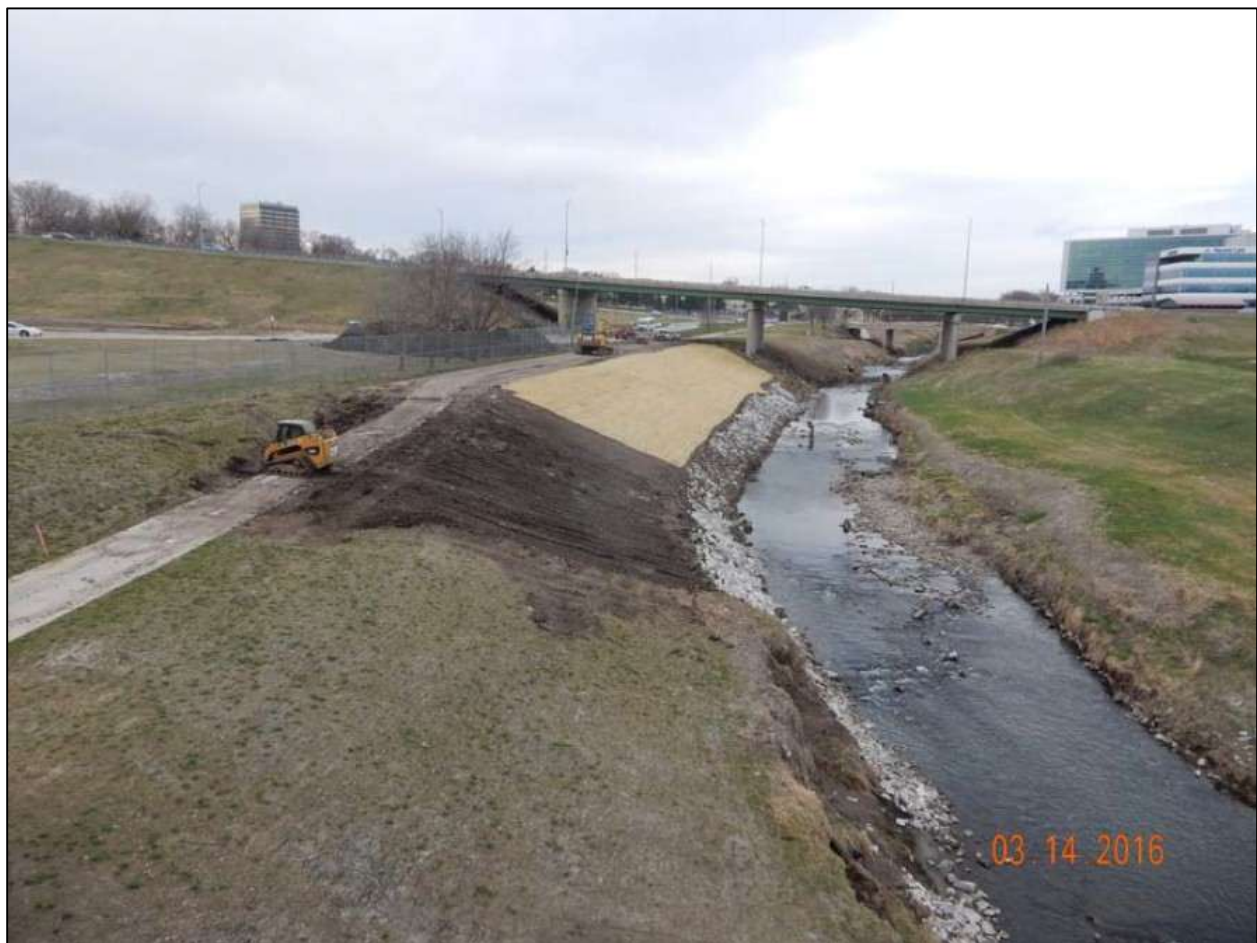
Figure 4. Successful Bank Stabilization of the Little Papio Channel by the Papio NRD
