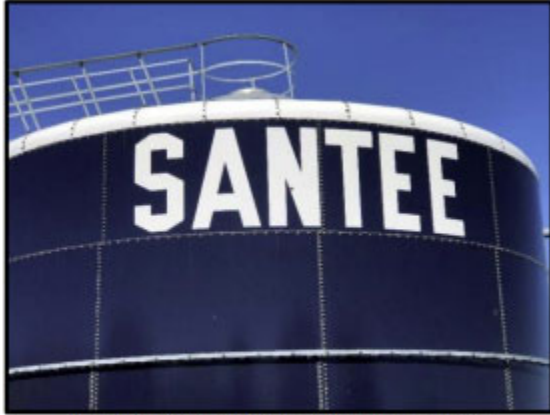
Picture 1: Village of Santee Water Storage Tank.
