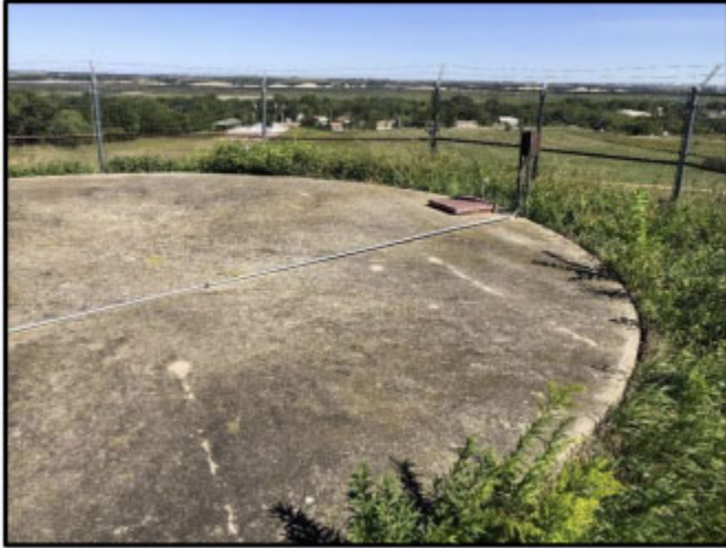
Picture 4: Exterior of 60,000 gallon below ground storage tank.
