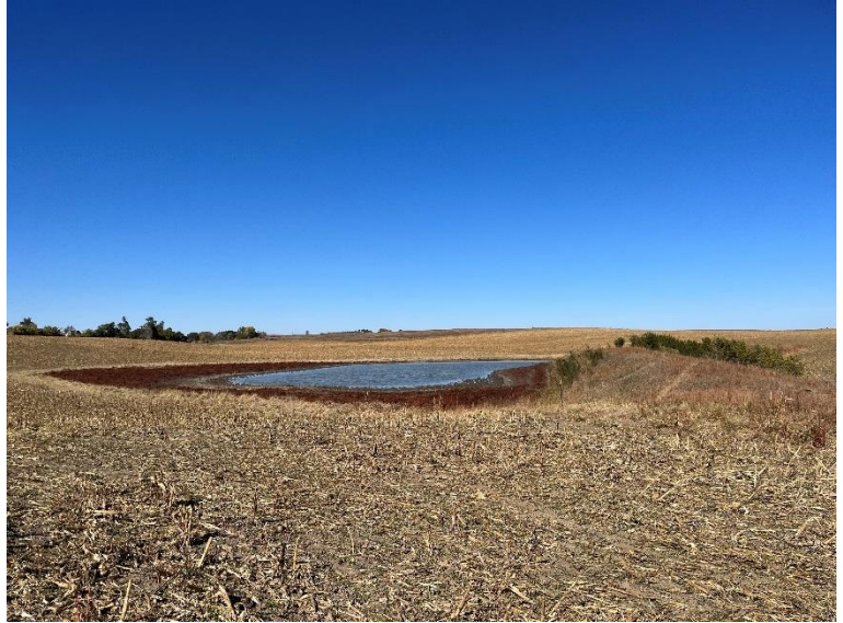
Picture of the Red Cloud Dam in 2022 (Credit: JEO Consulting Group, Inc.)
