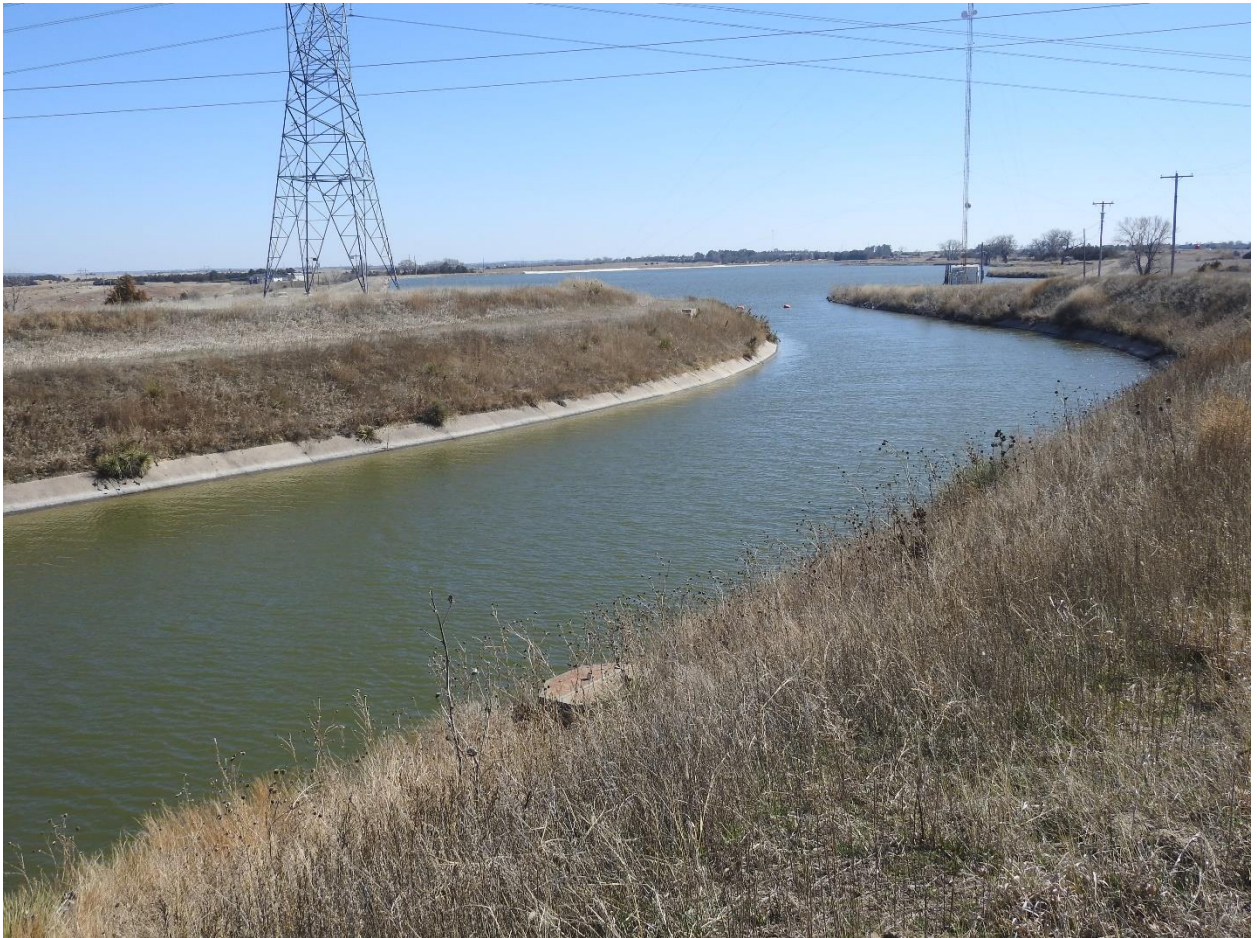
Figure 5 – Facility Forebay looking South Near the Penstock Inlet
