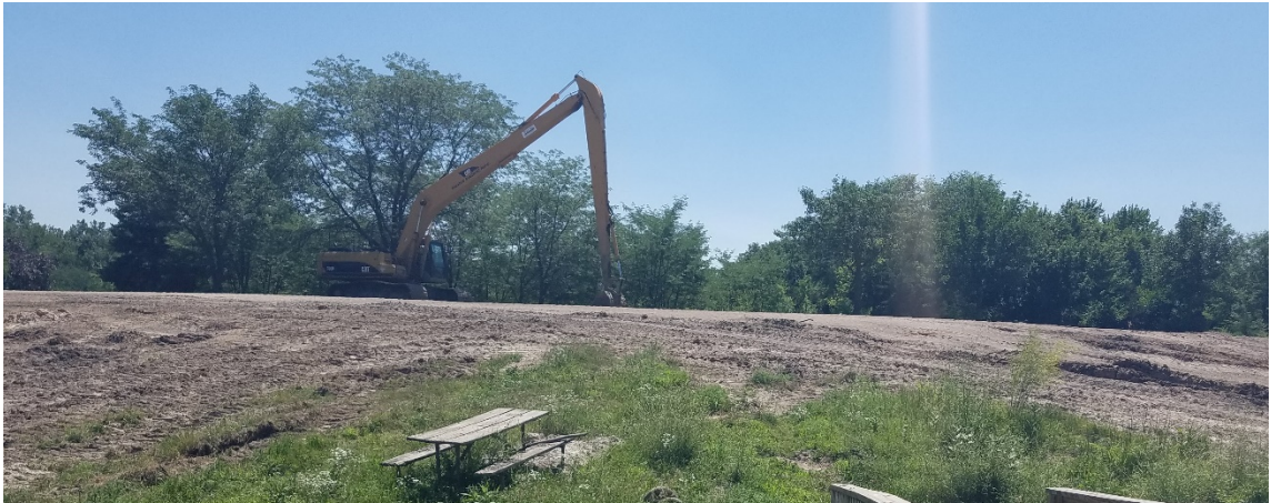
Figure 13 – Use of Excavator to Remove Sediment from a Waterbody (Crystal Lake)
