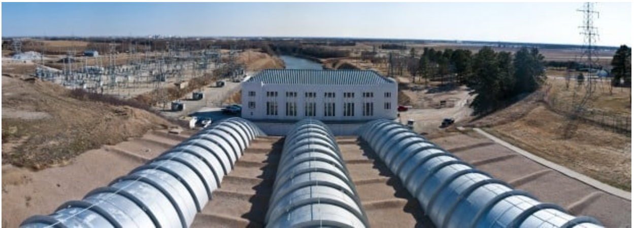
Figure 10 – Columbus Powerhouse Penstocks 7
