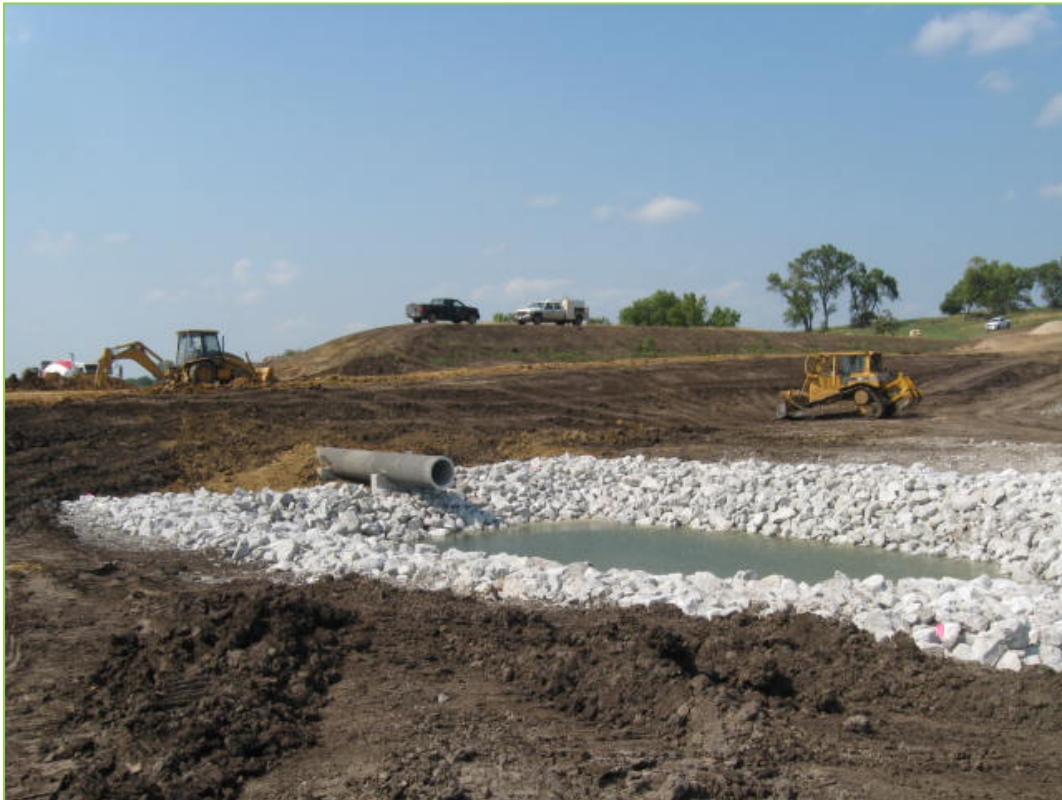
Image 9 Dam rehabilitation, Nemaha NRD
