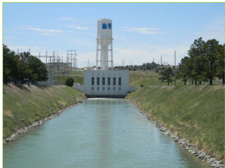
Image 5 Nebraska Public Power District, North Platte, Nebraska.
