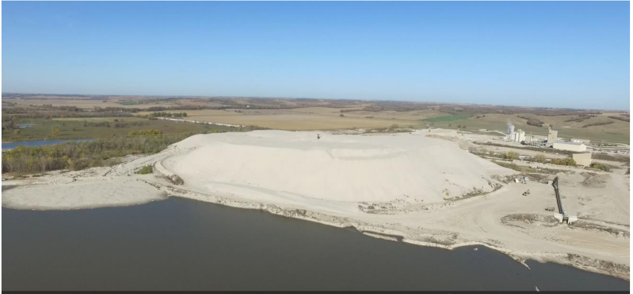
Figure: Sand Pile at the Head Gate
