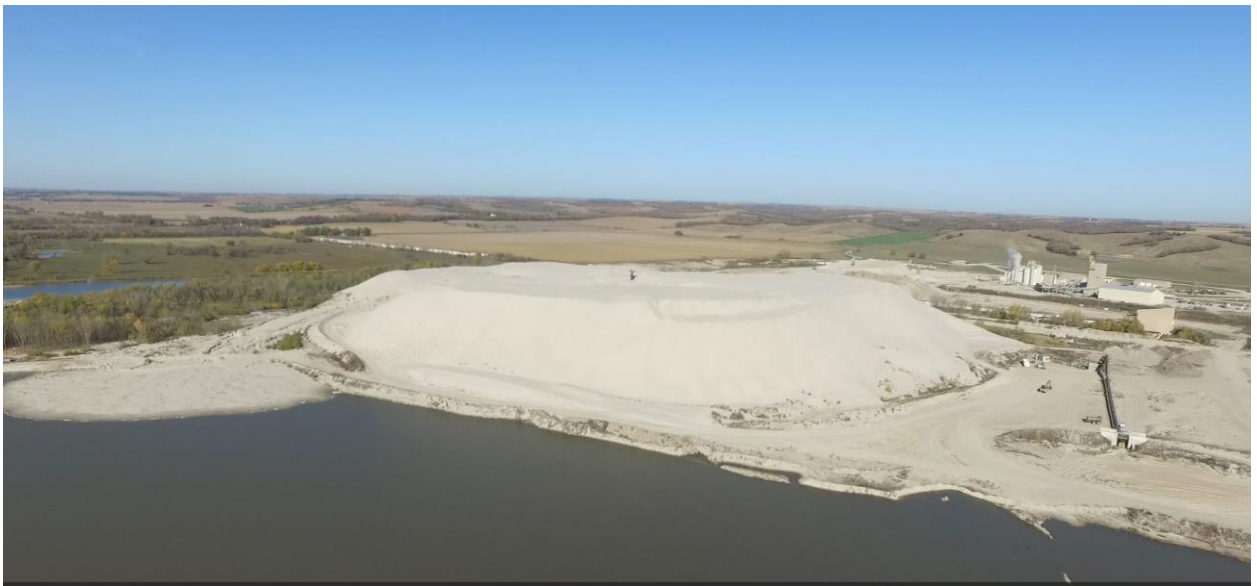
Figure: Dredged Sand Pile at the Headworks
