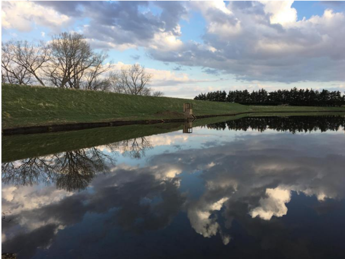
Little Indian Creek existing watershed structure example.
