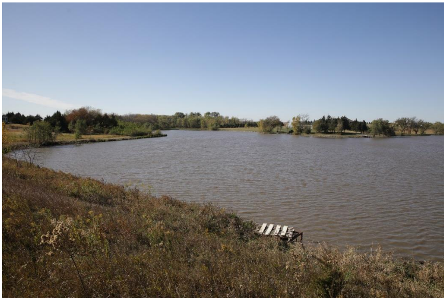
Little Indian Creek existing watershed structure example.
