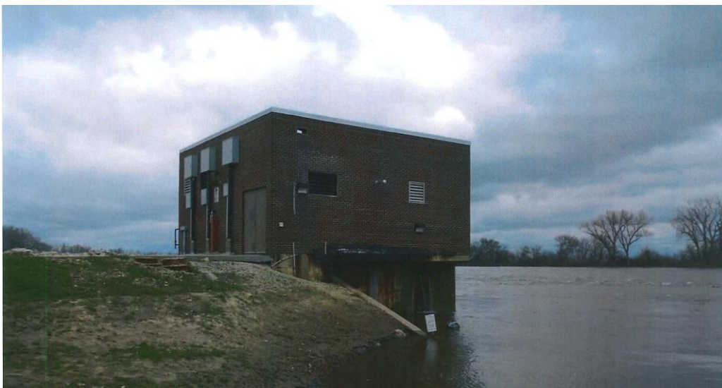
Figure 3 The Blair's water intake pump house on the Missouri River looking upstream.
