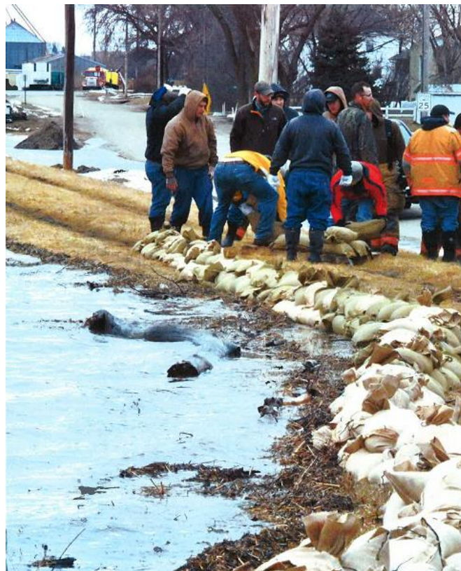
March 2019 – Volunteers place sandbags as floodwaters rise to the top of the levee system.
