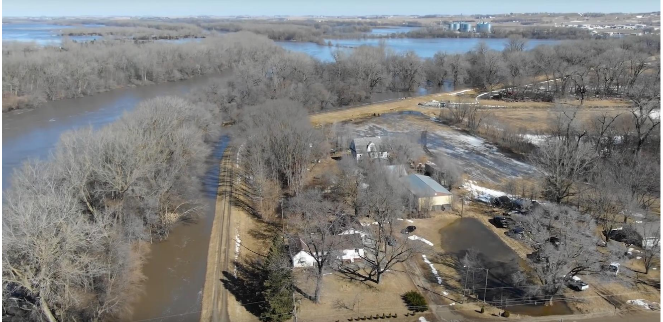
March 2019 – Elkhorn River floodwaters and existing levee at West Point looking north.
