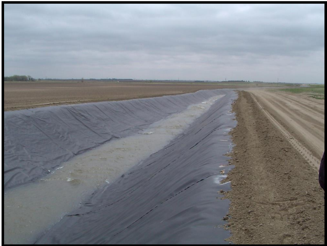
Figure 5. E67 Canal membrane-lined section: beginning of first fill.
