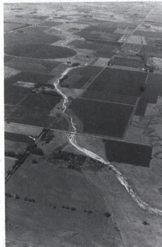
Silver Creek Flood Control Project located in Merrick County
