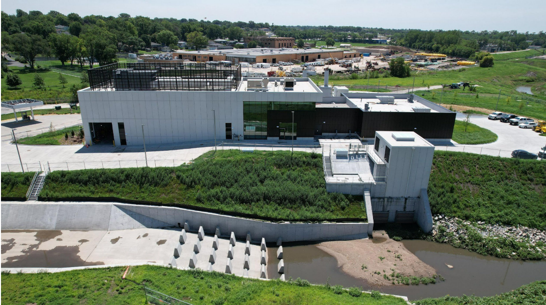
Aerial View of Saddle Creek RTB from North – July 2023
