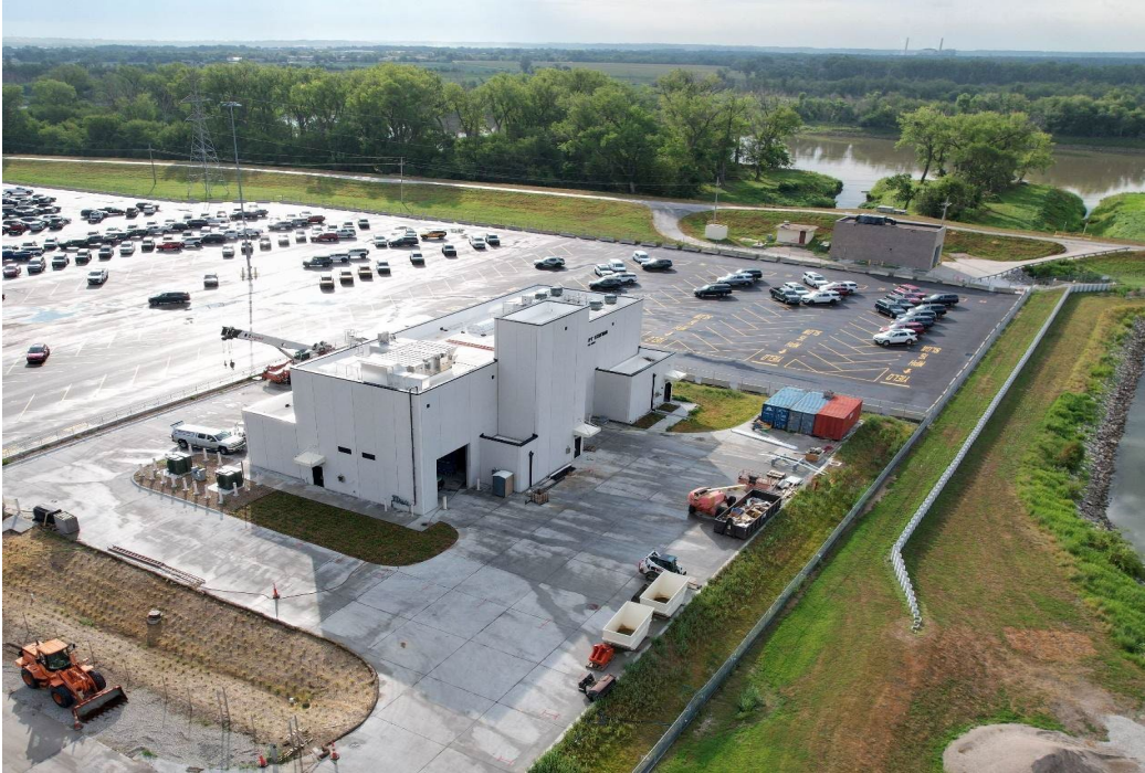
Aerial View of the Riverview Lift Station Project
