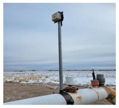
The following picture shows the digital "FlowCom" meter head that replaces manual, odometerstyle meter heads.
