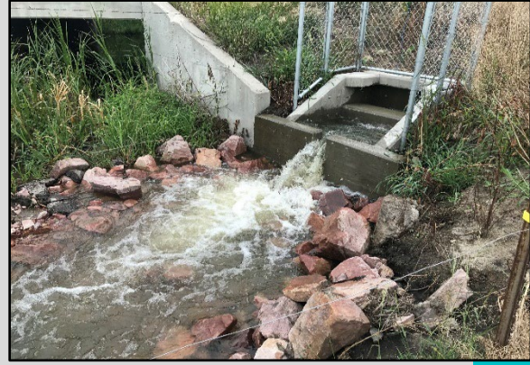
Surface Water Outlet Structure
