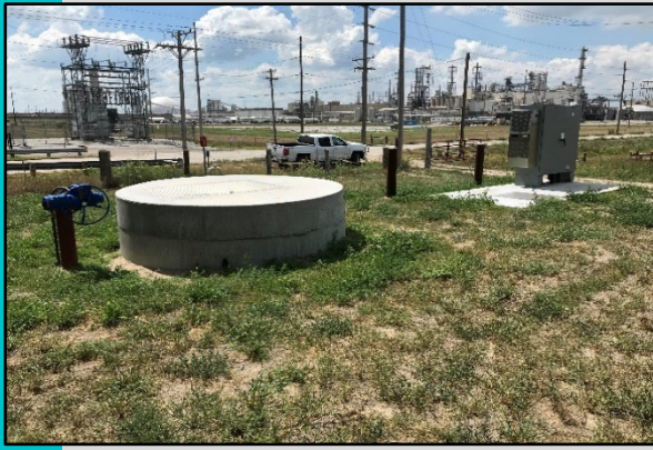
Surface Water Intake Structure
