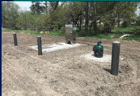
Auxiliary Well Structure
