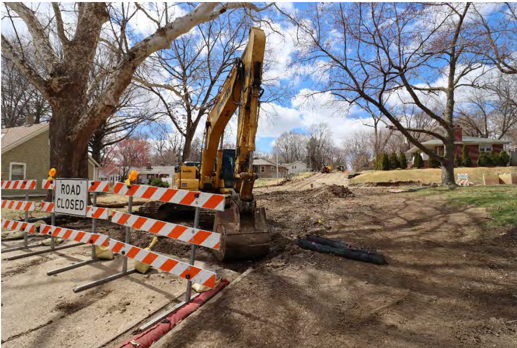
Figure 13 - PCN 210 Construction April 2022
