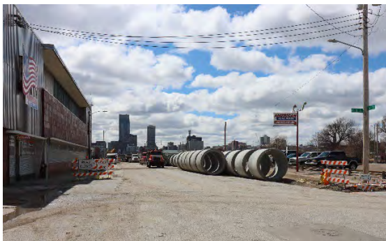
Figure 1 Material Storage for Nicholas St Phase 3B in April 2022
