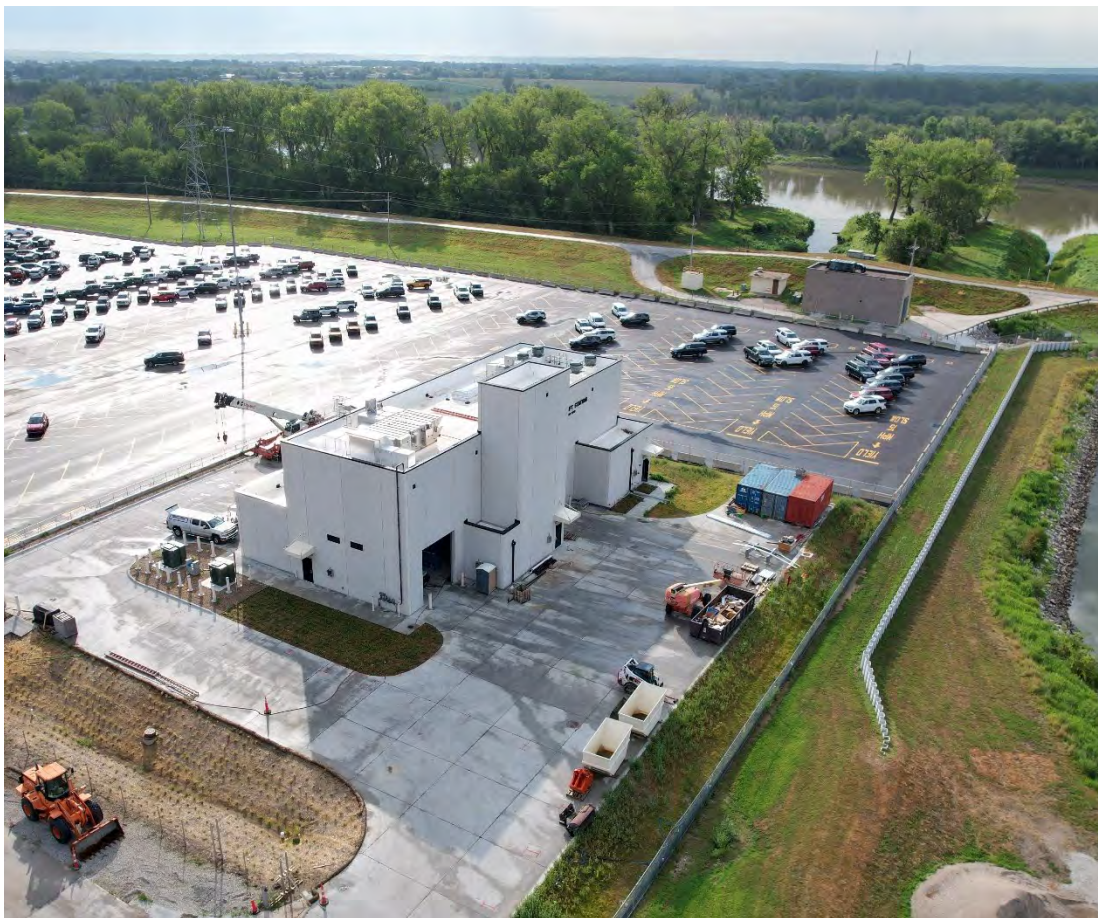
Figure 3-7. Riverview Lift Station August 2022 (Courtesy of Multivista)
