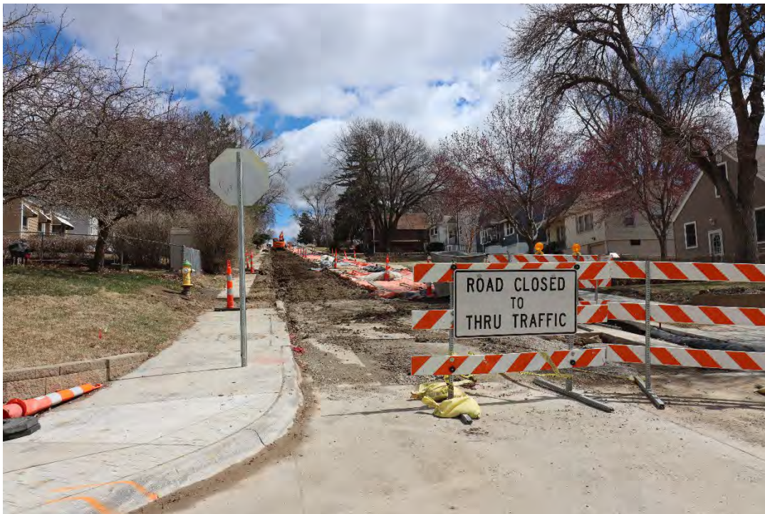
Figure 12 - Construction in the CSO 203 area in April 2022
