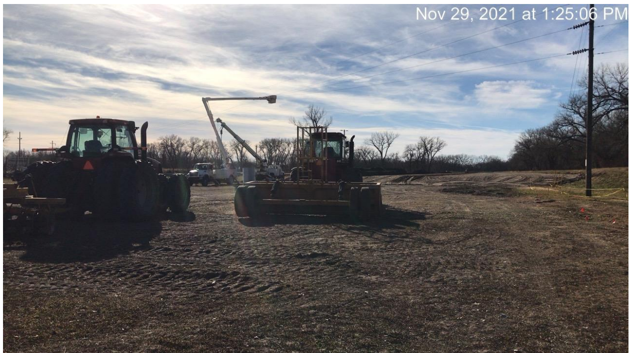
West Point Levee Seepage Berm Construction: Power Pole Relocation
