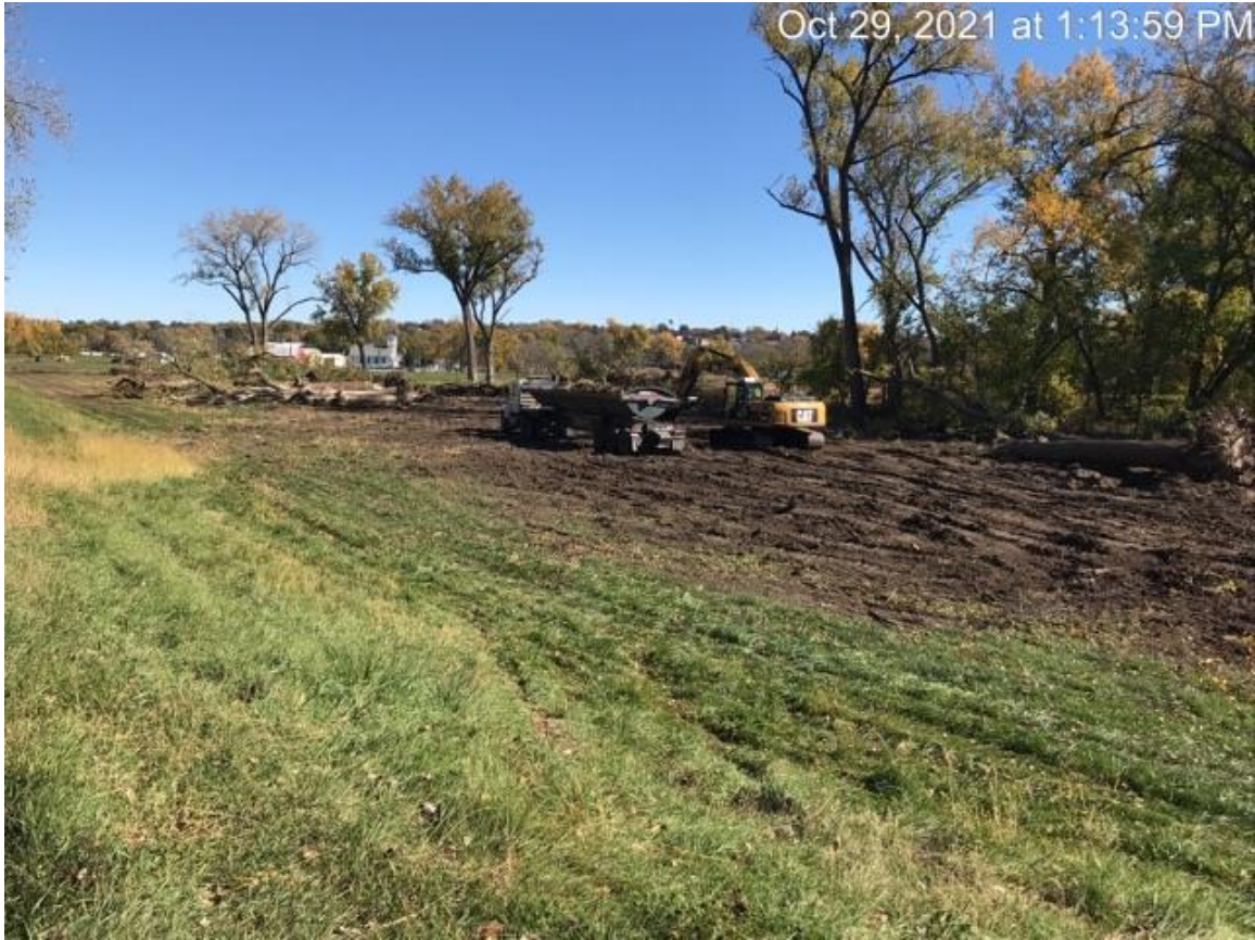
West Point Levee Seepage Berm Construction: Preparation & Tree Removal
