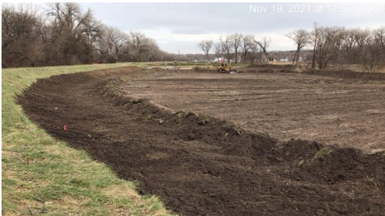
West Point Levee Seepage Berm Construction: Preparation & Topsoil Stripping
