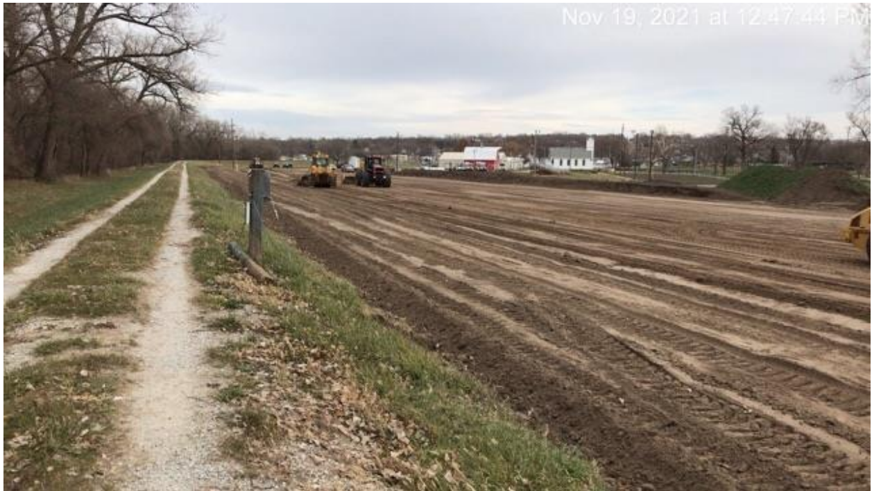
West Point Levee Seepage Berm Construction: Sand Seepage Berm Grading
