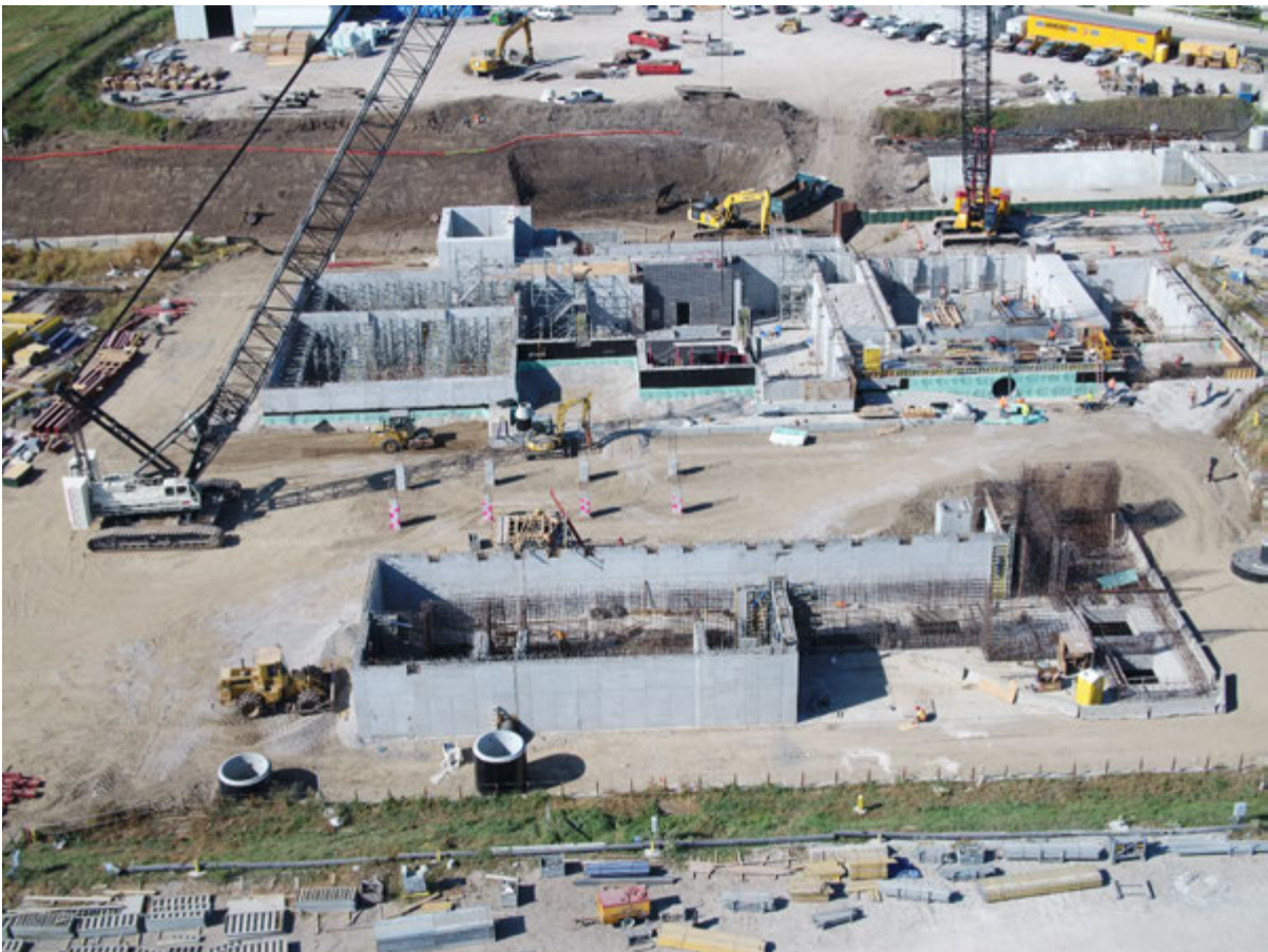
Figure 1 – Saddle Creek RTB Site Construction (October 2021). Chemical Building, Operations Building, and Headworks facilities toward the top of the picture. Dewatering pump station, flow meter vault, and other ancillary facilities toward the bottom of the picture.
