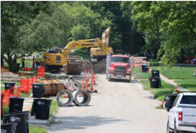
Figure 2. Construction on the CSO 203 project, July 2021
