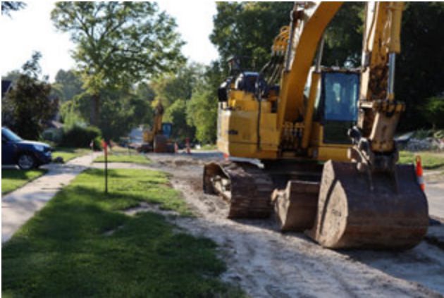
Figure 1. Construction on the CSO 203 project, September 2021
