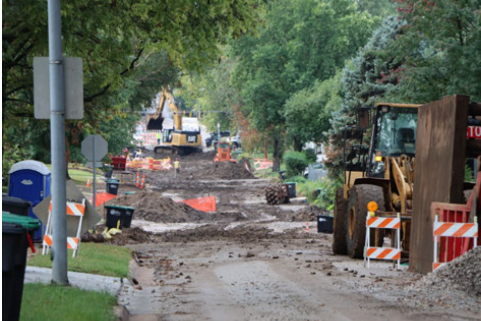
Figure 1. PCN 210 Construction September 2021
