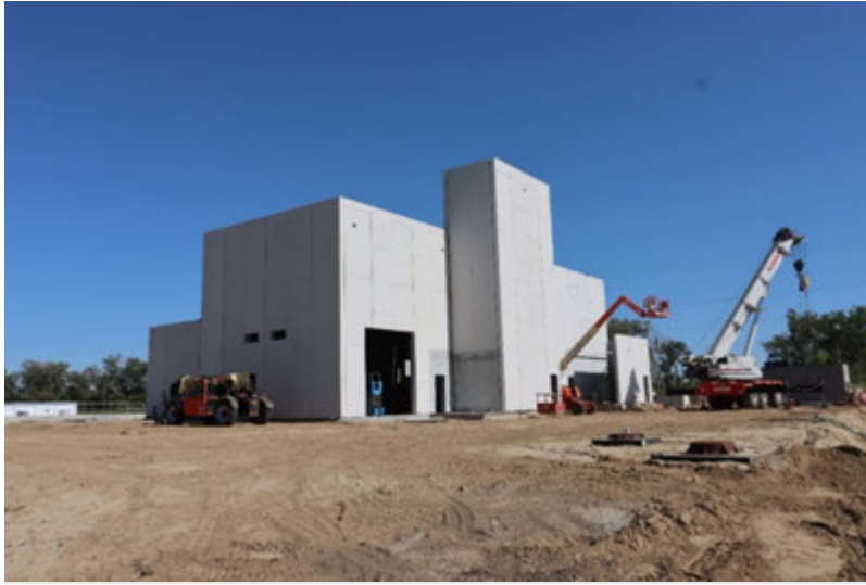
Figure 3-13. New Riverview Lift Station Construction Following Installation of Pre-Cast Concrete Walls
