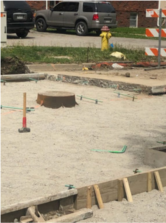
Figure 2. Paving preparation for intersection at North 60th Avenue and Taylor Street.
