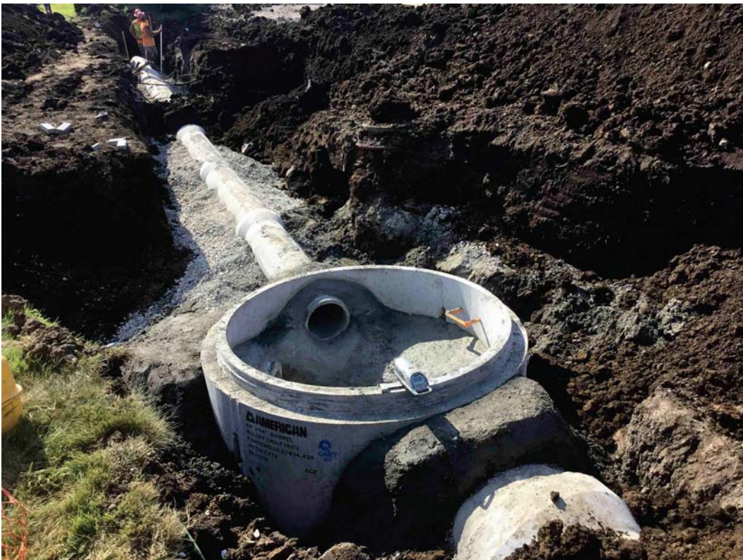
Manhole and Storm Sewer Construction in Fontenelle Park
