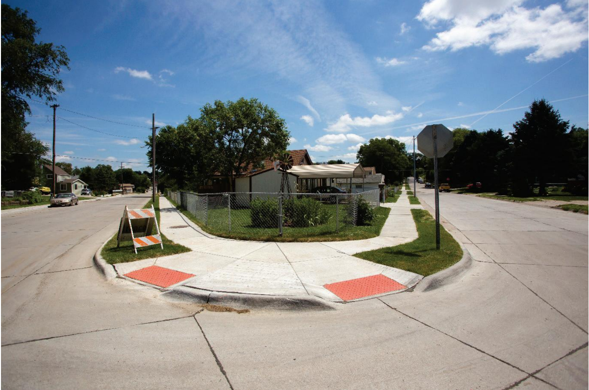
New curb and gutter and ADA compliance ramps
