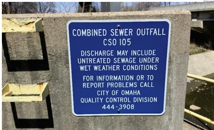
Figure 3-3: CSO 105 Outfall Sign
