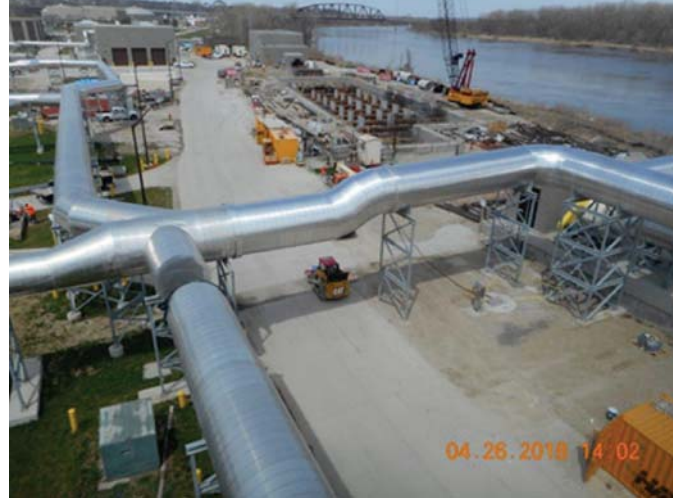
Figure 4-4: MRWRRF Improvements under Construction
