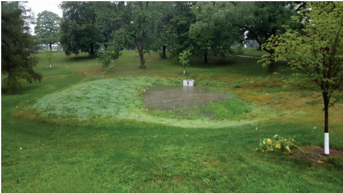
Stormwater in Hitchcock Park green infrastructure
