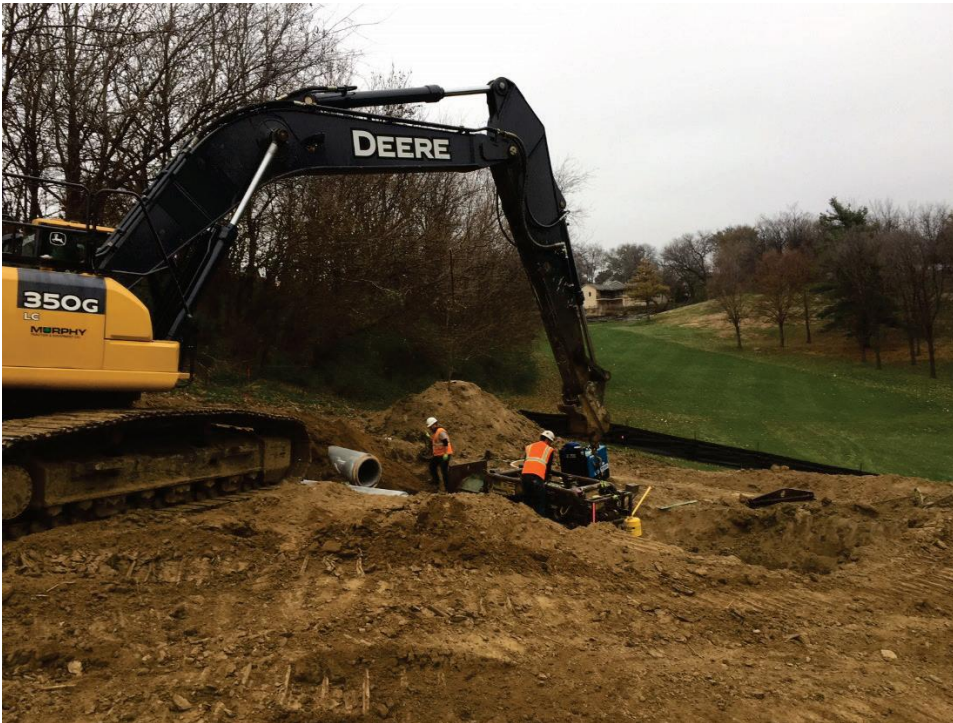
Storm Sewer Construction in Spring Lake Park Golf Course
