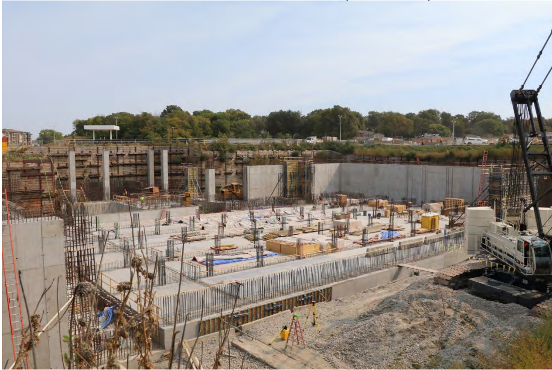
Saddle Creek RTB CSO 205 New Diversion and Outfall Channel Improvements, Sept. 2020
